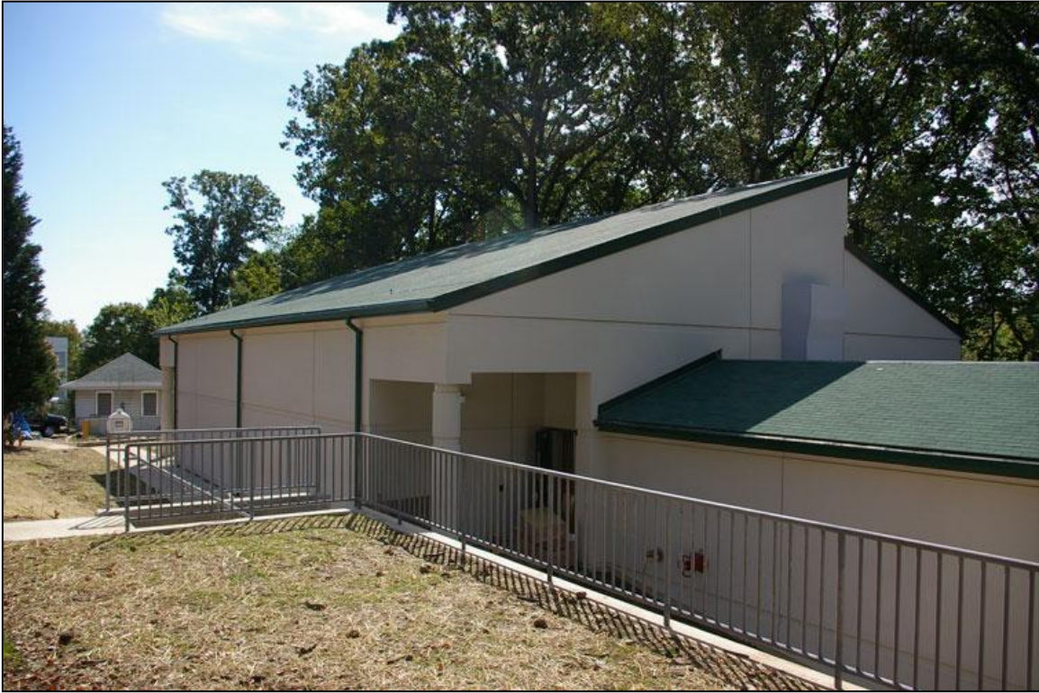
Figure 12. New clock building.
